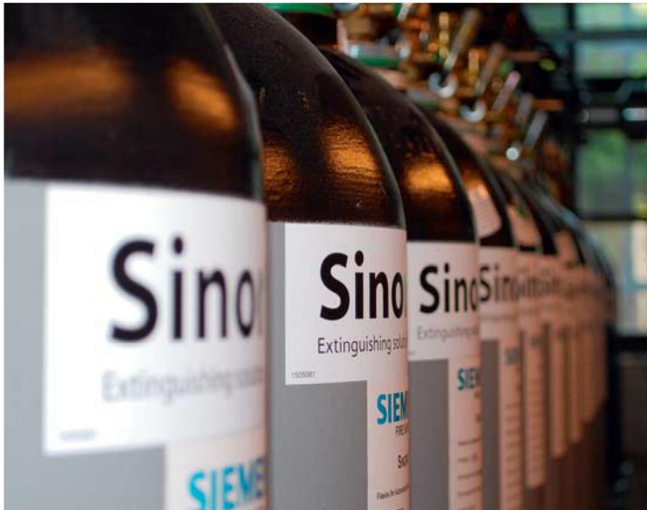
Depending on the application, nitrogen, argon or carbon dioxide is the optimal extinguishing agent.
