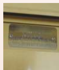
conformity mark fire rated
